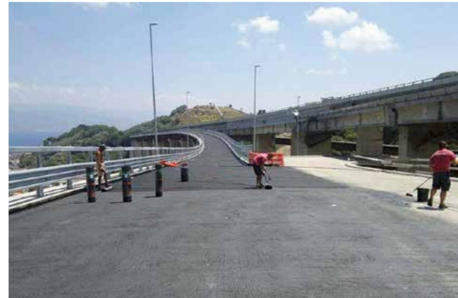
Preparing the installation layer with a primer for bituminous membranes. Using bituminous membranes on road surfaces allows to increase the durability and resistance of road surfaces, reducing maintenance costs.
