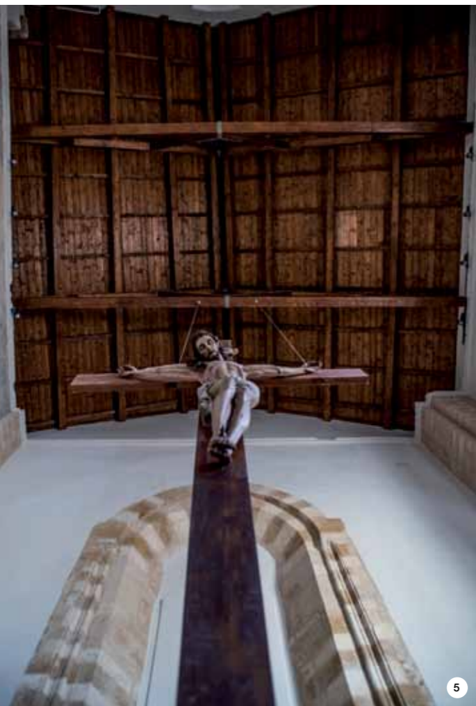
1. MAPE ANTIQUE F21 super-fluid binder was injected through small tubes using low-pressure pumps to consolidate the stone structure.
