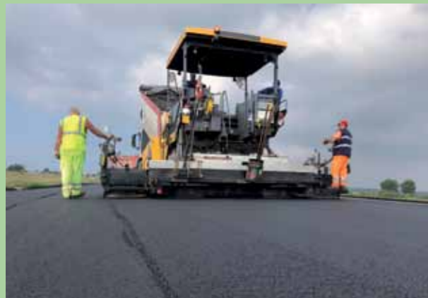
FROM LEFT ON. Mapei has developed new admixtures for creating new bituminous conglomerates that allow substantial amounts of road asphalt to be recycled.
