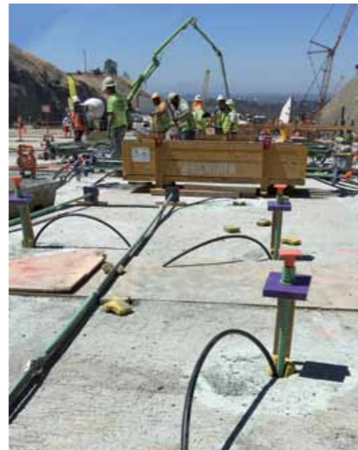
ABOVE. PLANIGROUT 755 was pumped in to fill the voids between the pieces of rebar and the outer wall of the core.
