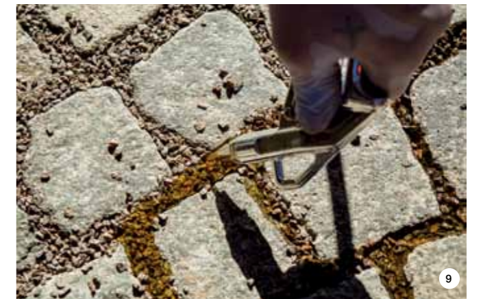
the installation bed, blocks and filler in the gaps between the blocks. 8. After vibro-compacting the paving, the installation bed and filler between the blocks settled and the spaces in the gaps between the blocks were topped up again with crushed porphyry. 9. MAPESTONE JOINT solvent-free polyurethane binder was poured manually into the gaps using Zème equipment.
